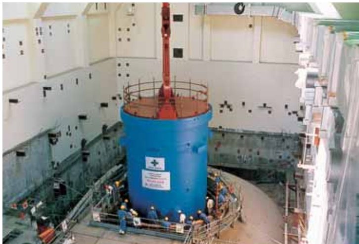
1994 Installation of the Reactor Pressure Vessel
