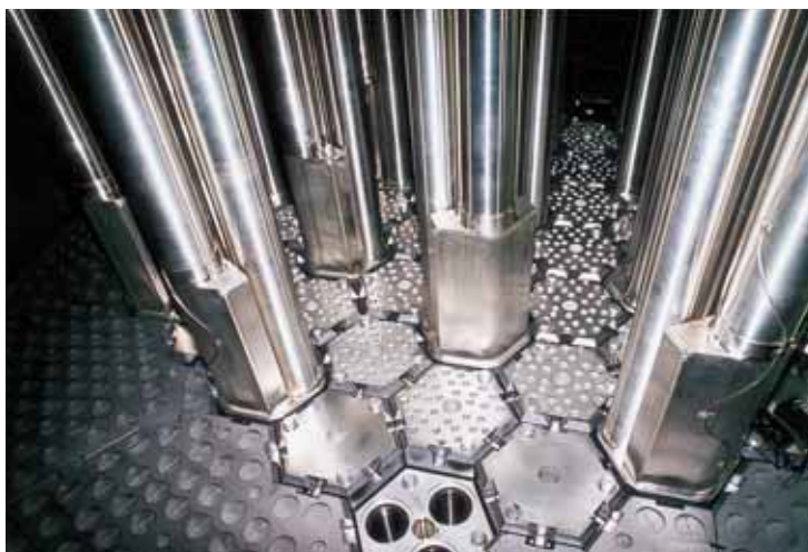
1996 Inside of the Reactor Pressure Vessel
