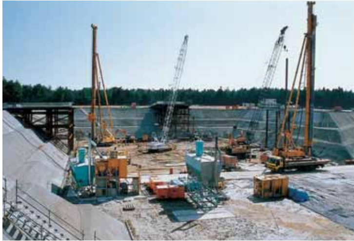
1991 Start of HTTR construction
